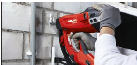
Conduits and light-duty pipes
