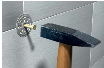
Flush hammer set installation
